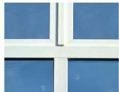
CC-Effect® on PVC after 2 years weathering
